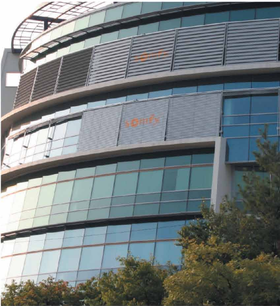
Louver and EVB installation with Somfy motors at the Korea Institute of Construction Technology (EVB installed on the 4th floor, Louver installed on the 5th floor)
